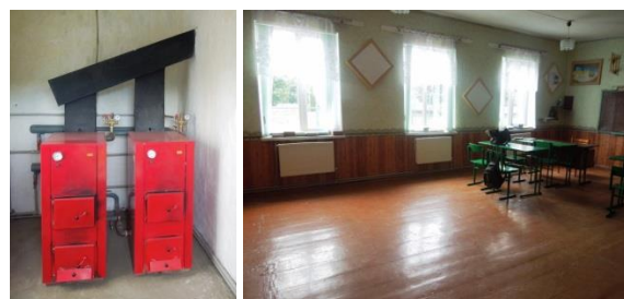
New boiler, new batteries and insulated windows in a school
