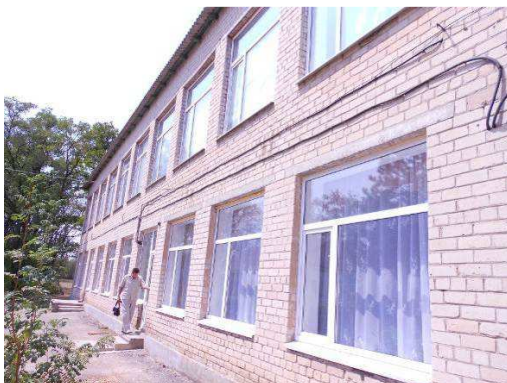
CO of Korniivka village (Zaporizka oblast) completed their micro-project on energy saving in a local school
