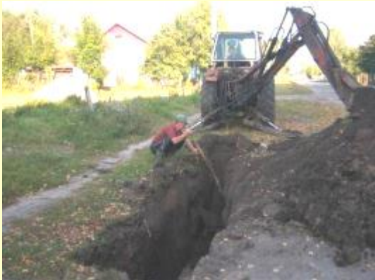
Capital repairing of water supply system in v.Verba (Rivna region)
