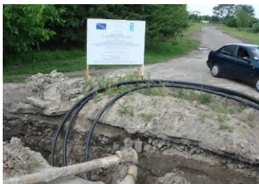
Temporary display of 'Repair of water supply system', Yerkivtsi village of Kyivska oblast
